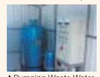
▲Pumping Waste Water for Reuse
