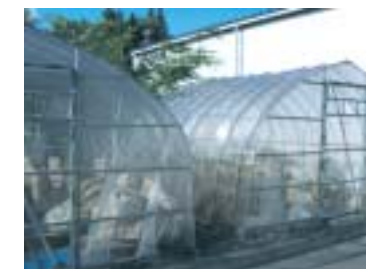
The plastic Greenhouse for drying sludge
