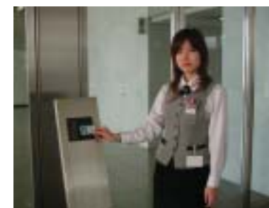
Building access control system
