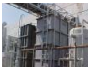
Pure water storage tank
