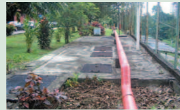
Upper side of the plant
