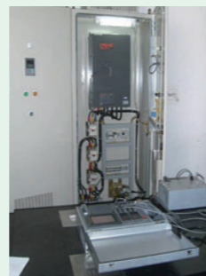
Variable speed drive unit
